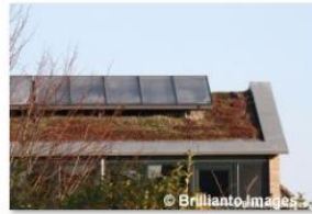
green roof solar hot water panel -Schönberg Germany (C) Brillianto.JPG
